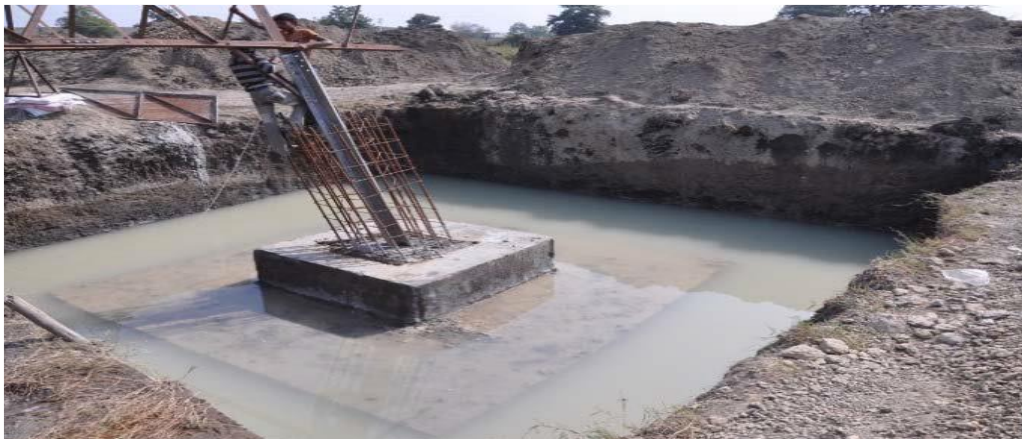
Figure 15 Tower-base and foundation
