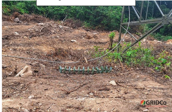
Damaged Conductor & Cables
