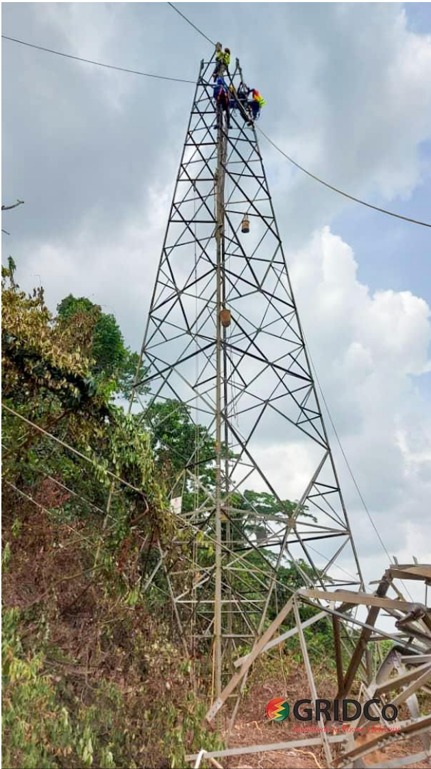
GRIDCo Engineers working to restore the Line
