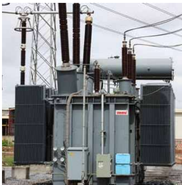
One of the 330 kV 200 MVA transformers in service at the Volta Substation
