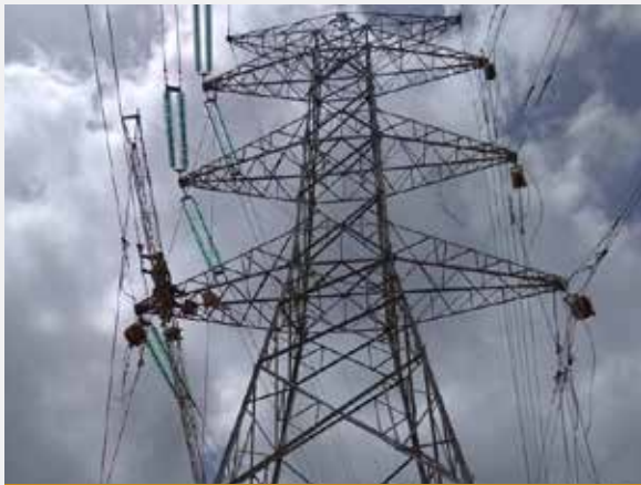
Conductor Stringing Works In Progress : Aboadze- Prestea 330kV Transmission Line
