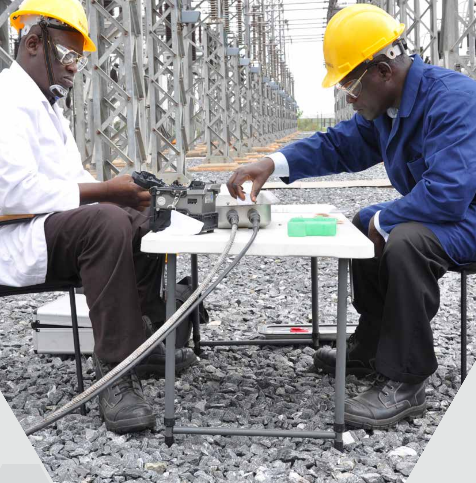
Splicing of OPGW and Approach Cable for Smelter II- Enclave Power Transmission Line at Smelter II Substation.
