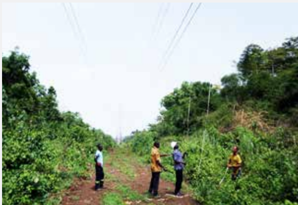
Vertical Clearance checks on the 161kV Mim-Juaboso Transmission Line
