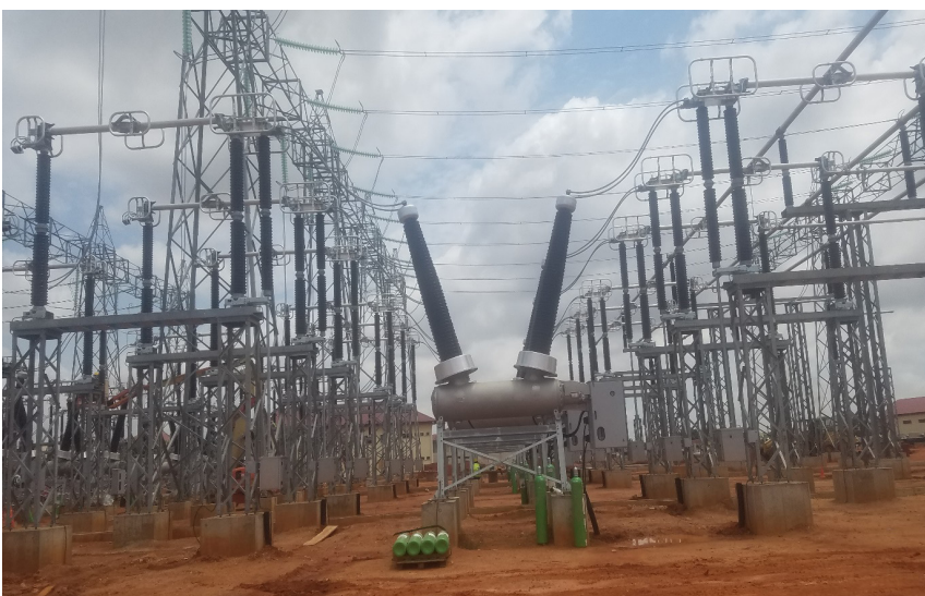
330kV Circuit Breaker installation works at the Pokuase Substation
