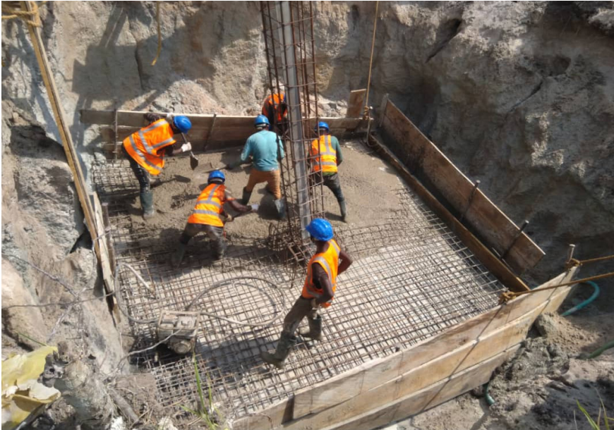
330kV Kumasi-Kintampo Transmission Line – Tower foundation works at Ejisu- Konkor
