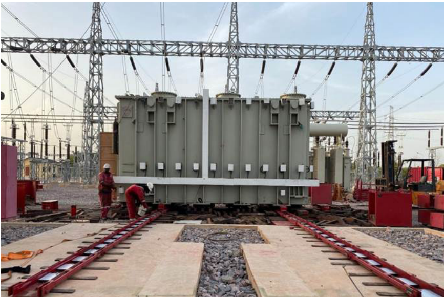
Set up of Delivered Autotransformer on its pad at the Bolgatanga II substation
