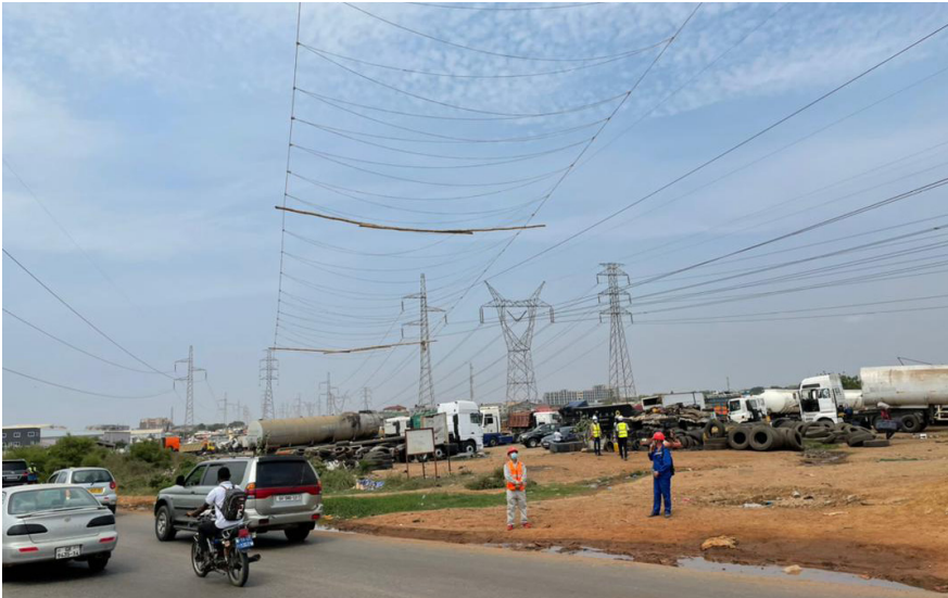
Contractor on Volta-Achimota Line installing a web (netting) at road crossing before stringing at major road crossing.
