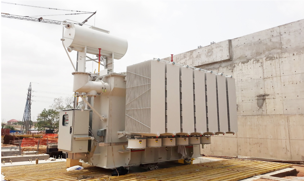
Kasoa Bulk Supply Point – Delivery of Statcomm and Power Transformers
