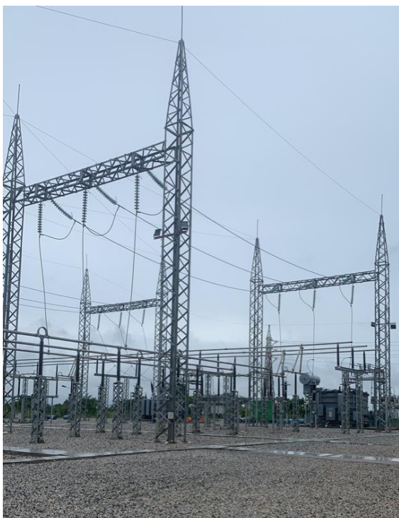
The completed 34.5kV Berekum Substation
