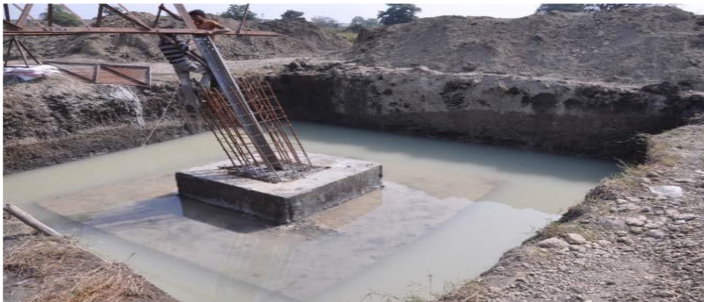
Figure 8 Tower-base and foundation
