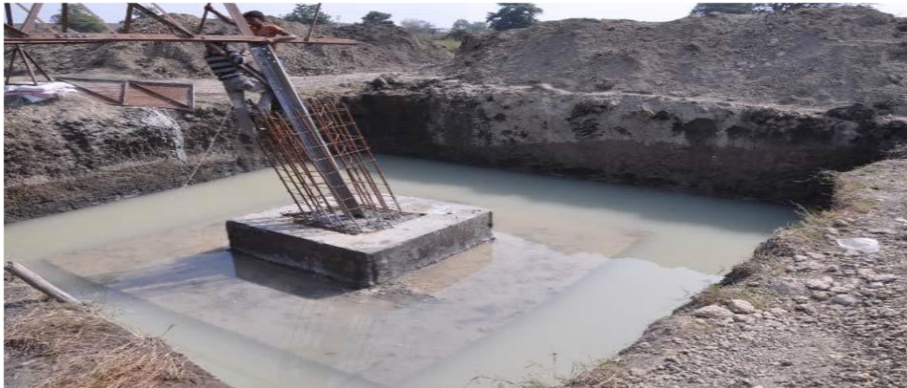
Figure 8 Tower-base and foundation
